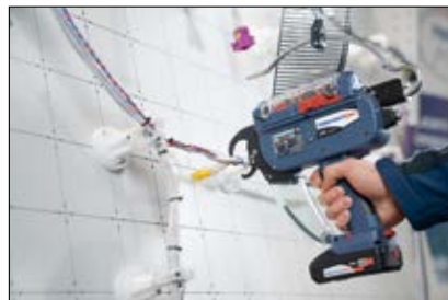
Operated by battery with cable ties on a reel from overhead suspension
